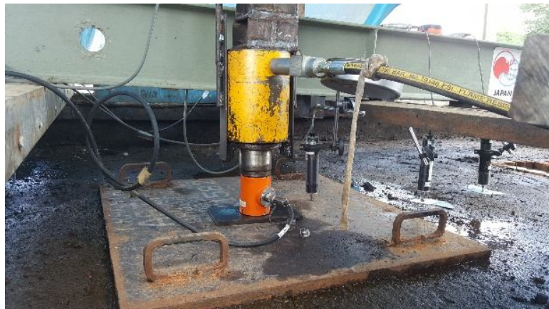
Fig. 4 Axial loading test of soil
